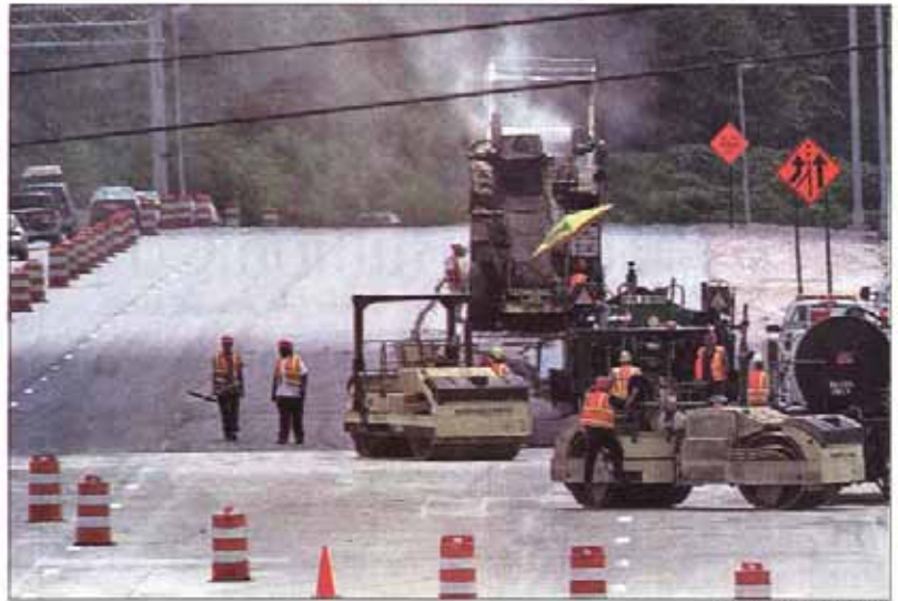
Workers pave part of Interstate 40 in downtown Knoxville in this July 2001 photo. The high price of asphalt means state and local governments are pursuing fewer road projects these days. Bruce Wuethrich, senior director of engineering and public works for Knox County, said the county has not had to sacrifice capital projects — the building of new roads or major reconstruction projects that generally cost more than $50,000. Instead, it has scaled back maintenance projects in subdivisions.
